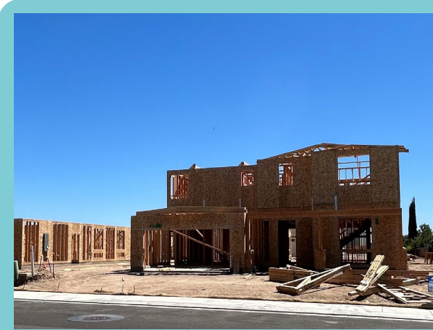
Construction of Keyes 19 homes
